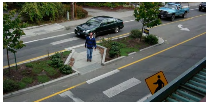
FIGURE B-11: CROSSING ISLAND ANGLED TO ENCOURAGE PEDESTRIAN AWARENESS OF TRAFFIC ON THE ROADWAY ABOUT TO BE CROSSED (PHOTO BY BRUCE LANDIS)
